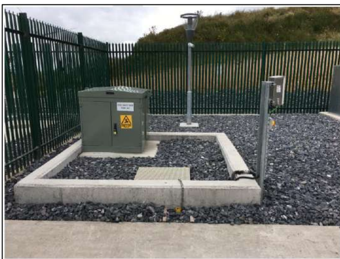
Figure 9. Location of CCTV Cameras on Lighting Column
